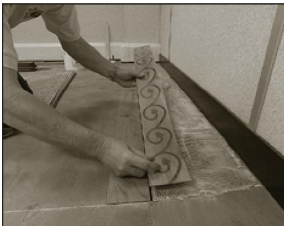
Setting out for border installation
