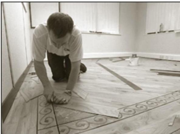
Installing border and perimeter tiles
