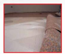
Move to the opposite side and carry out the same process. Once the first strip is complete, move onto the next, adjacent strip ensuring and checking that each strip is tightly butt-joined with no overlaps and NO GAPS. Immediately roll the underlay with a medium weight 45kg stand up roller prior to the adhesive curing. Roll the entire floor in both directions to ensure optimum adhesive transference.
