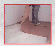
3. INSTALLATION - Adhering DAMTEC® acoustic underlay to substrate.
