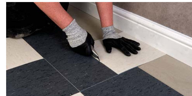
Figure 5 Measuring using an overlapping tile
