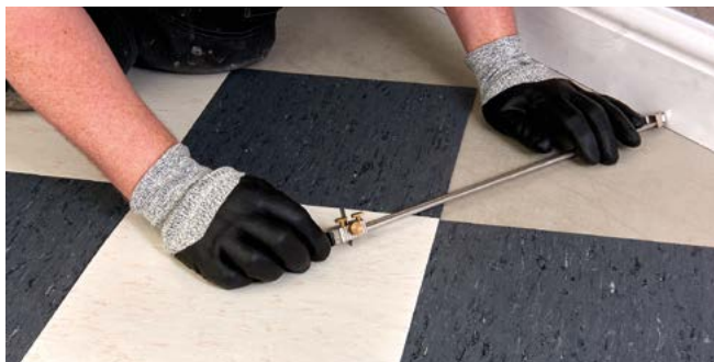
Figure 9 Cutting the tiles using a scribe (diagonal cut)
