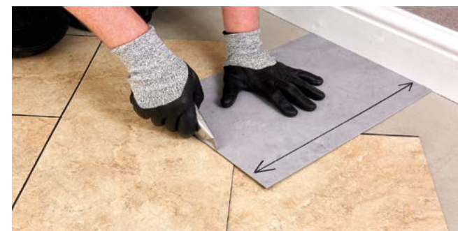
Figure 9 Cutting the perimeter tiles (diagonal cut)
