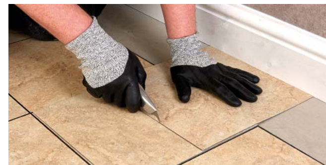
Figure 6 Measuring using an overlapping tile
