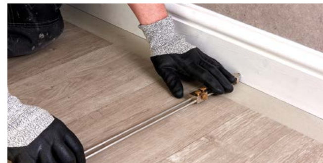
Figure 2 Scribing the wall profile
